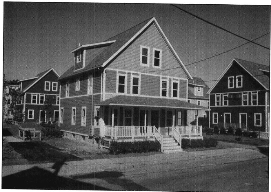
Lucerne Gardens, Boston, under construction
