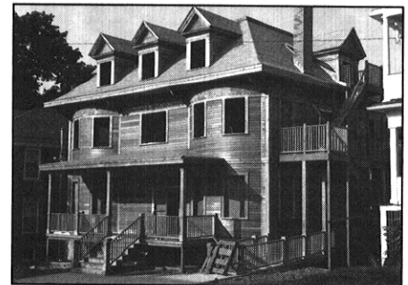
123 Crawford Street, Roxbury, after construction
