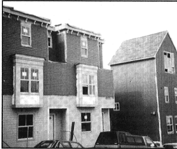
Fr. Walter Martin Cooperative, Boston, under construction
